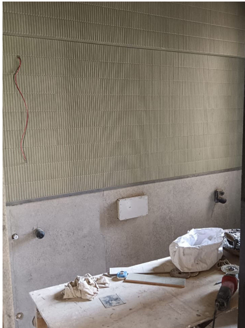
Tilework ongoing in bathrooms on site
