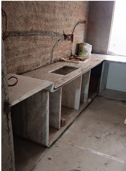
Carcass for kitchen and wardrobes being prepared on site
